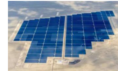
Utility Scale Solar
