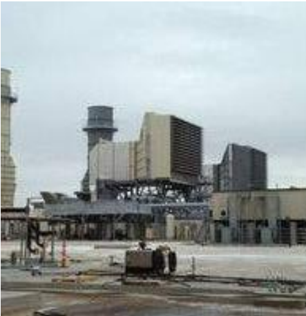
Xcel Energy’s Jones Station, TX.
