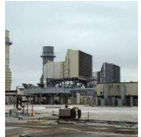
Xcel Energy's Jones Station, TX.
